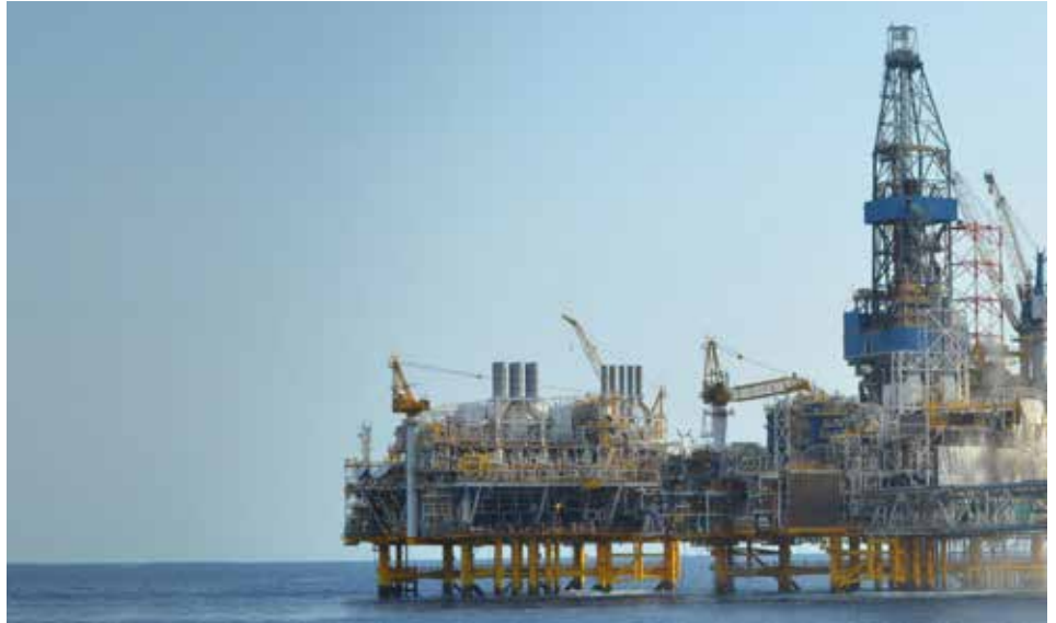
Drilling and production platform handling high-flow-rate gas wells with high condensate ratio offshore Australia.
