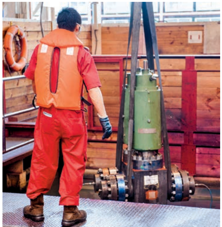
Hydraulic actuated gate valves being gas-tested
