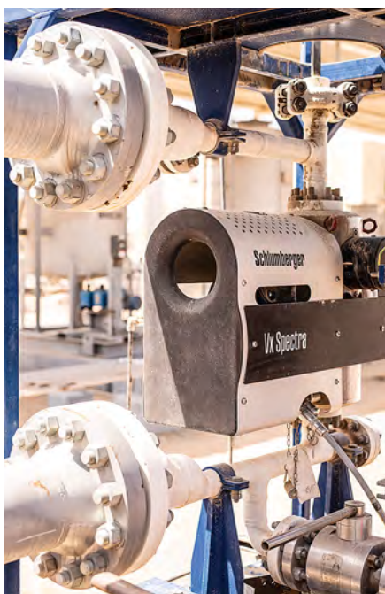
Fig. 4. Installation of the surface multiphase flowmeter in a Texas oil field.
