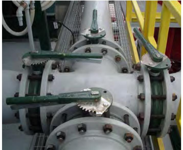
*Mud tanks require a large amount of butterfly valves to control mud traffic as this is a critical part of maintaining drilling operations.*
